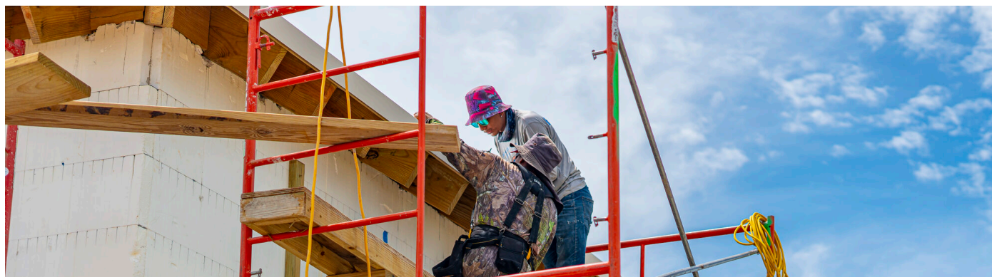
ICF wall construction.
